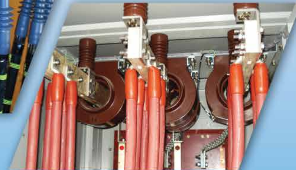
HV – TERMINATION WORKS (22 kV)
