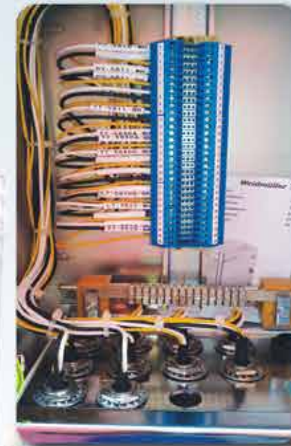
TERMINATION OF JUNCTION BOX
